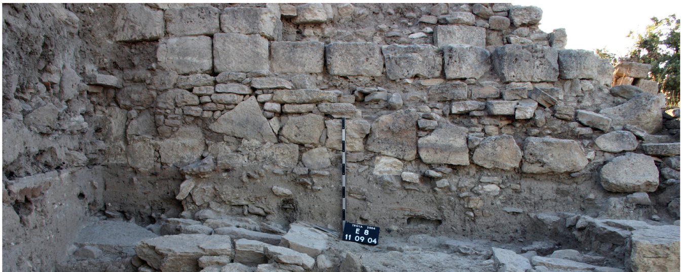
E. Room I. Division wall between Room I and Room H consisting of two orthostate courses above each other. The division wall is superposed by a Roman foundation made of ashlar blocks. (Dig 26169)
