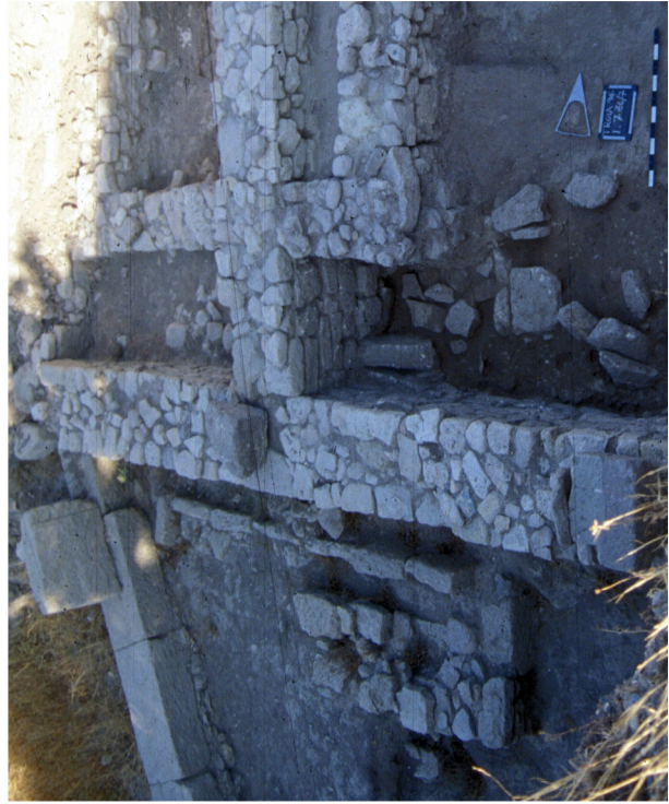
D. Possible disturbance responsible for discontinuity in VSF-1 north of the Hellenistic Wall (Dia 16582)
