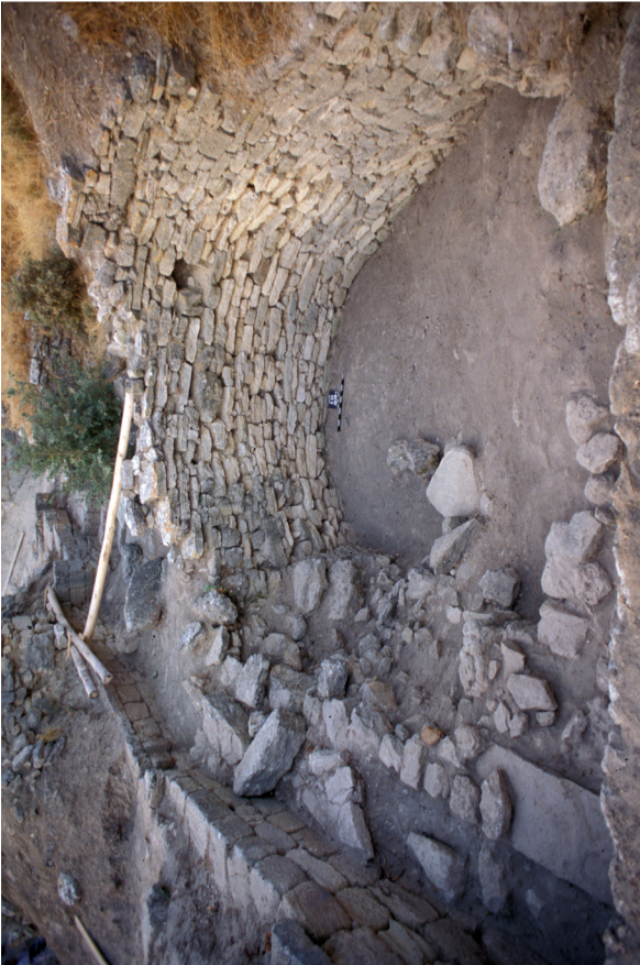
A. Well Bb inside the Northeast Bastion at the beginning of the Tübingen excavations, after the removal of the vegetation. View from the north (Dia 17584)
